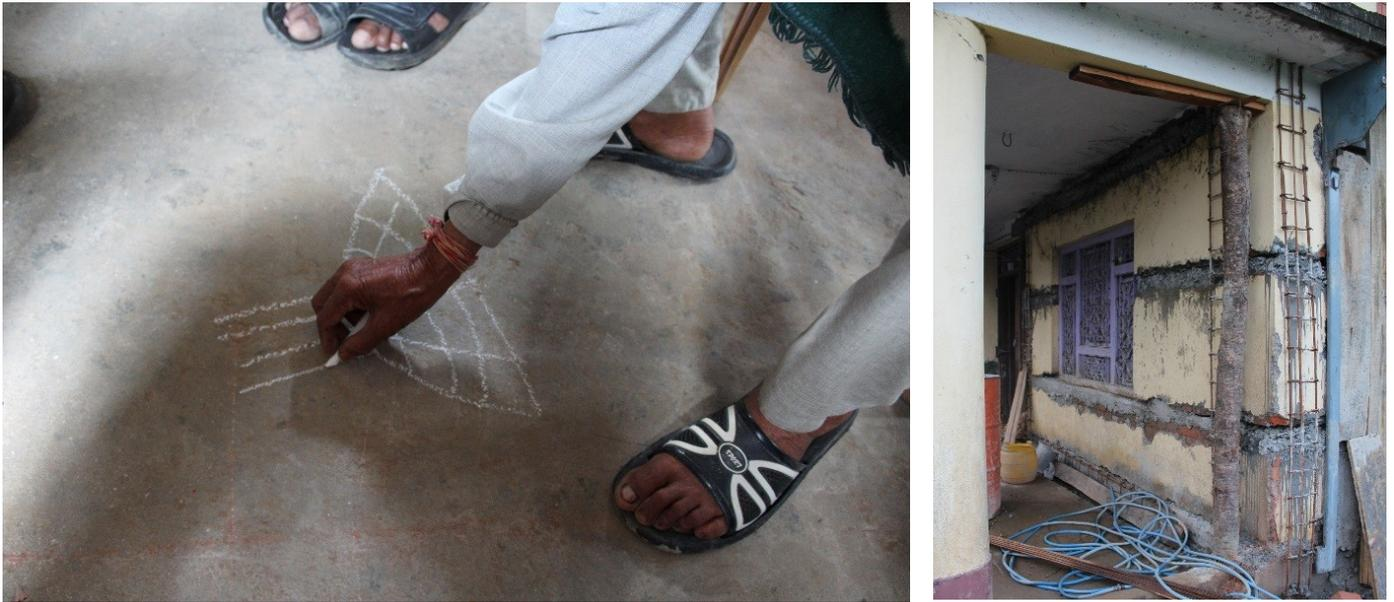
Figure 12. A mason in Bhaktapur drew how they now bent reinforcing steel into foundation footing, rather than simply cutting them at the foundation. The mason explained that he learned this technique as part of his school retrofit training. In North Kathmandu, houses near the school retrofit site were being retrofitted by adding bands and stitches two months after the event. The work was being carried out by local masons who had been trained to retrofit the school. Photo: R. Paci-Green/Risk RED
