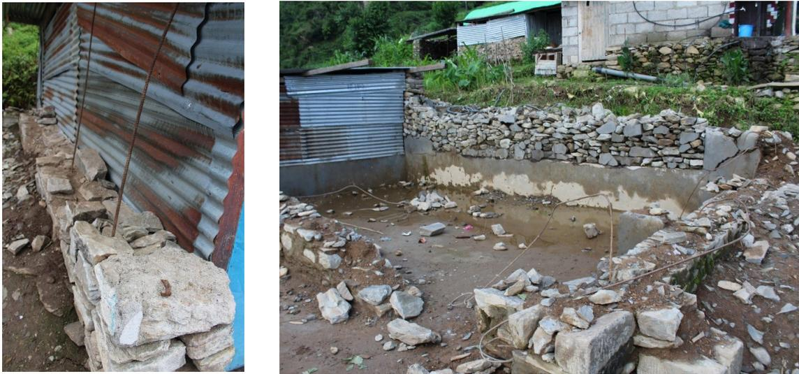
Figure 4. A Ministry of Education template design, which called for vertical rebar to be placed in stone walls, completely collapsed in every block assessed with this design. While now removed, after the earthquake, the classrooms were filled with stone from the collapsed walls. Photo: R. Paci-Green/Risk RED
